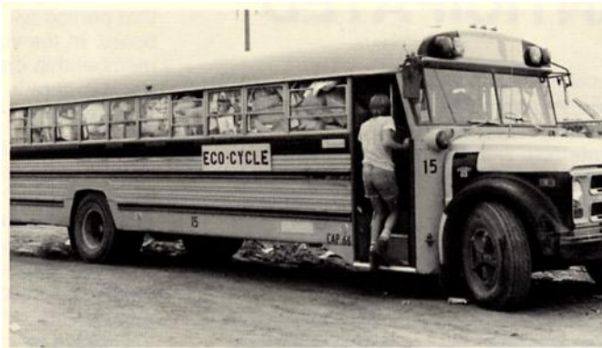
Eco-Cycle uses reconditioned school buses to move recyclables.
